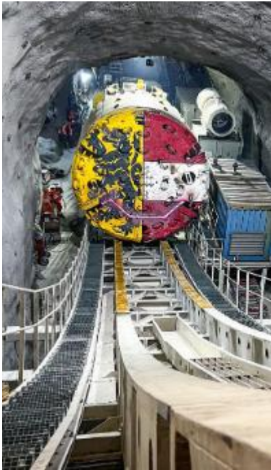
Figure 3. 5.8m diameter Gripper TBM assembled in horizontal position shortly before 50m vertical curve radius.
