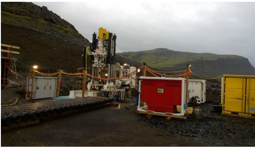
Figure 5. Herrenknecht VF 400 raise bore rig in use for the Búrfell II shafts.
