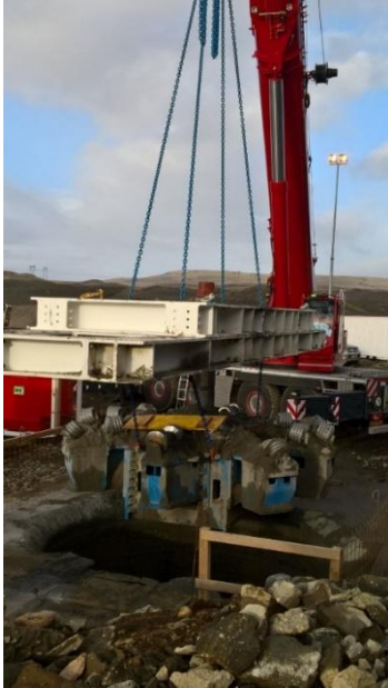
Figure 6. Herrenknecht VF 400 raise bore rig reamer head used for the cable shaft.
