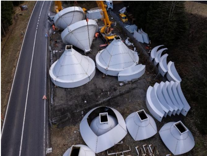
Figure 7. Assembly strategy requiring closure of highway lanes at night
