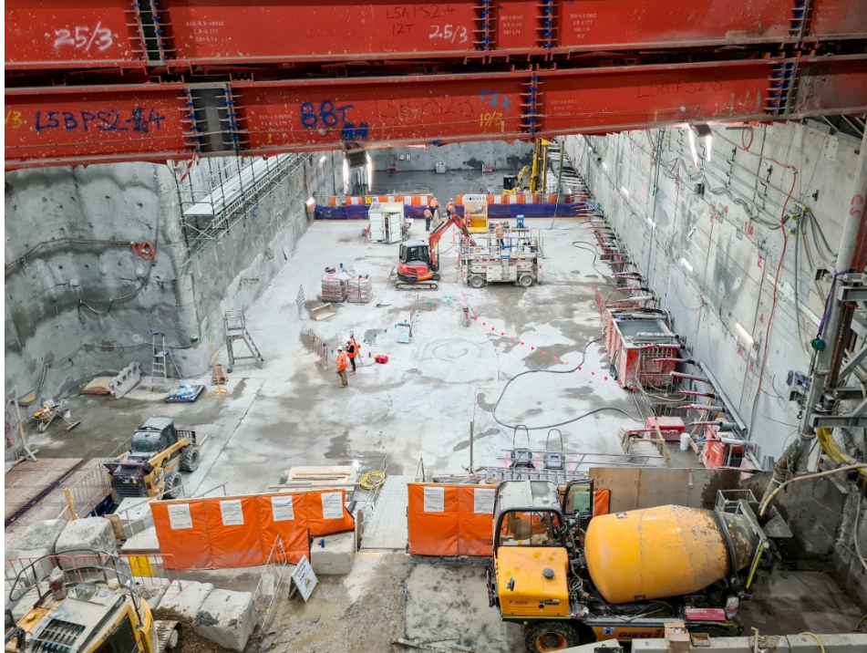
Figure 8. Construction Stage prior to stressing anchors
