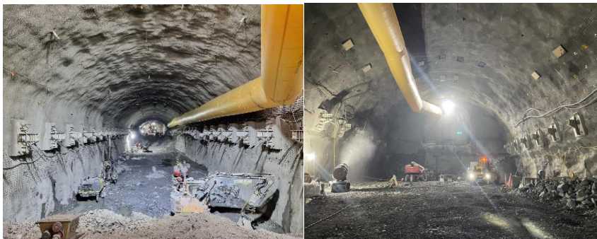
Figure 4. Stage 3 excavation of TH (left); Stage 3 excavation of MH (right)
