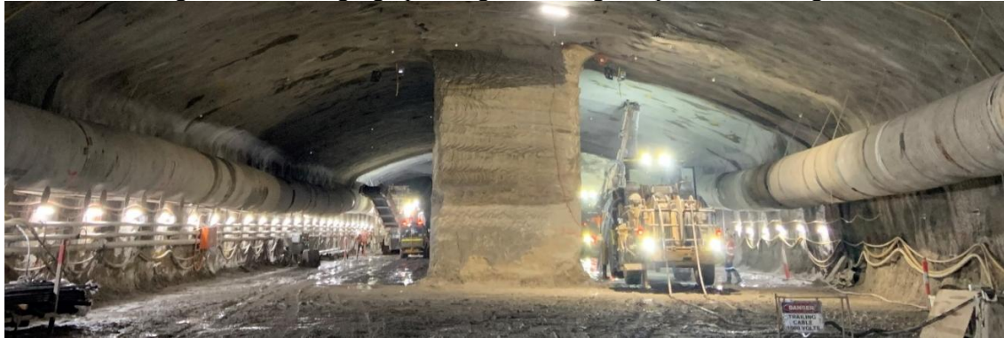
Figure 9. cavern under construction, showing a roadheader in heading 1 (left) and a bolting rig operating in heading 2 (right). The temporary central pillar (heading 3) is still in place.
