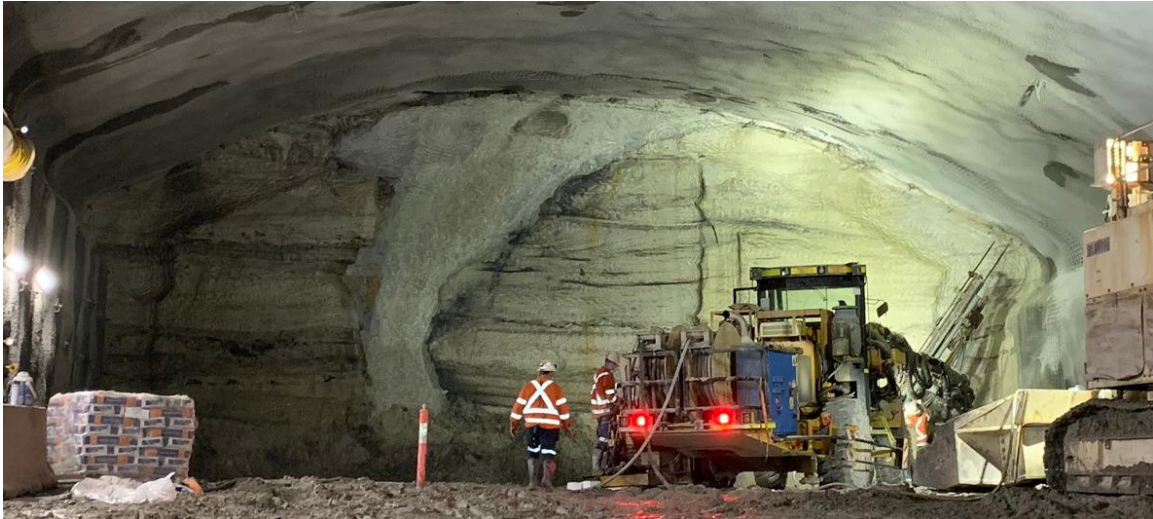
Figure 6. Dyke B encountered in the top heading of ventilation facility VF04.
