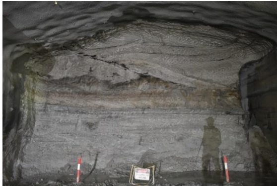
Figure 4. Fault 1 encountered in ramp adjacent to concrete replacement pillar of Cavern 5.
