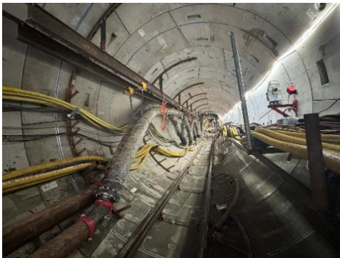
Figure 7. Muck discharge process with the slurry circulation system
