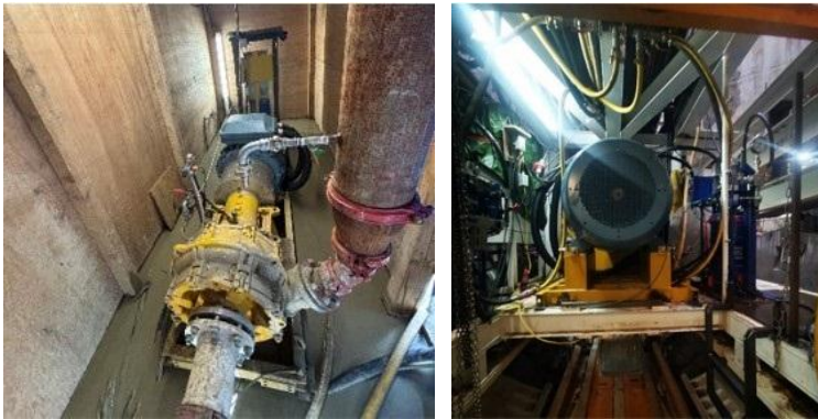
Figure 3. Slurry feeding and discharge pumps
