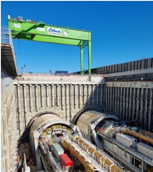
Figure 7. 550t capacity, 47m span gantry crane
