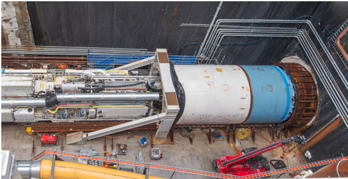
Figure 7. TBM backup gantry cradle, launch frame, temporary ring cradle and launch seal at the headwall
