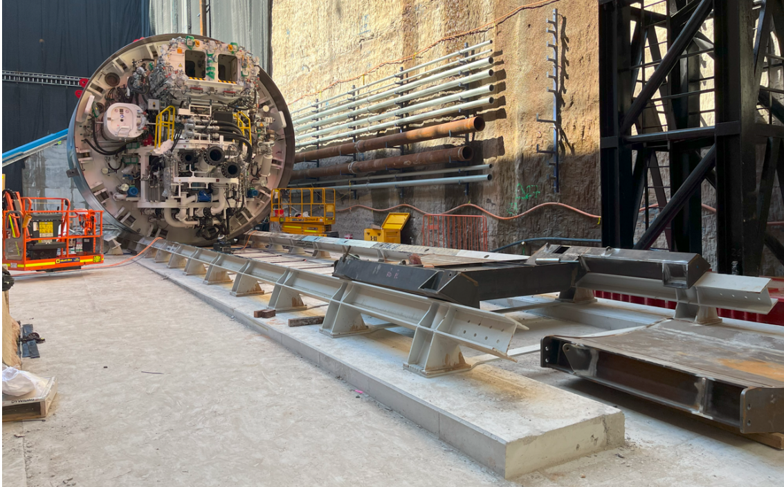
Figure 3. TBM shield during assembly on shield cradle, jacking dolly in foreground
