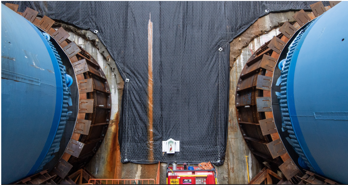
Figure 10. TBM launch seals at The Bays Station
