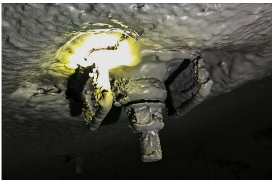
Figure 4. Membrane gap at bolt / shotcrete interface
