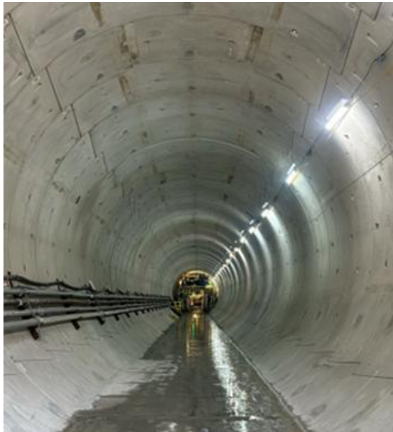
Figure 7. Completed segmentally lined tunnel
