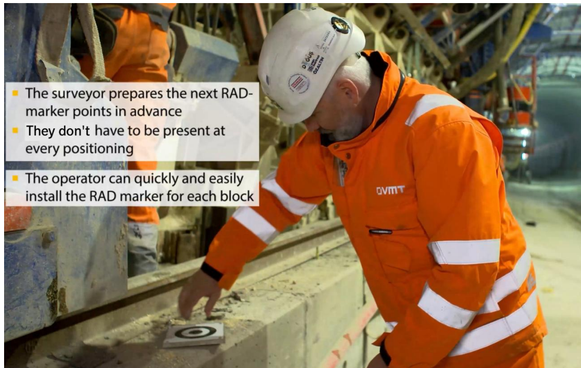
Figure 4. Production personnel screw in a RAD-marker to pre-coordinated survey “spigot”
