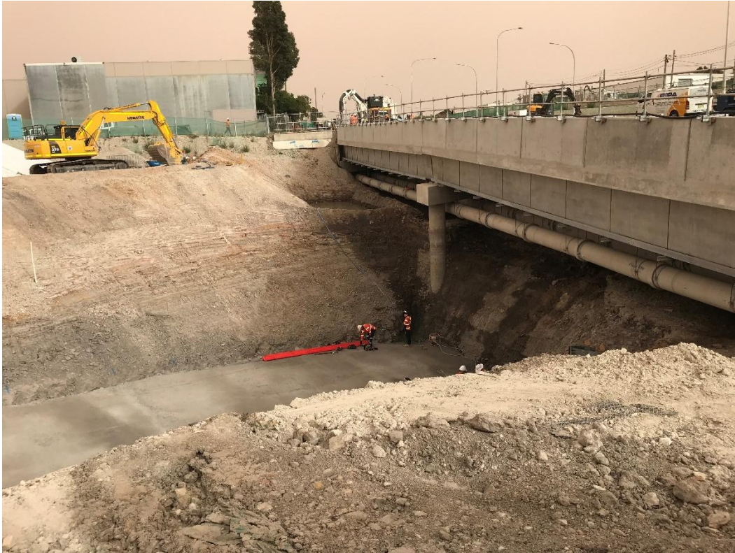
Figure 1 Existing cut and cover tunnel structure (southern end, photograph taken prior to stage 2 rock excavation works)
