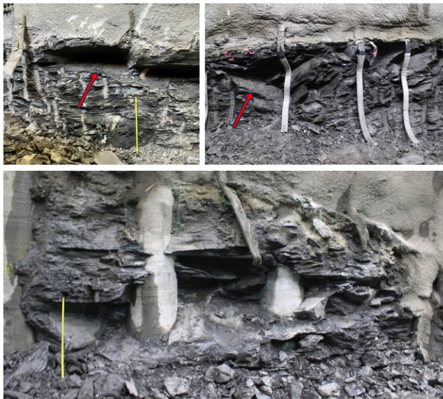
Figure 4. Typical wedges along mid angle defects in Ashfield Shale exposed during excavation. Wedge limited by piles (bottom).
