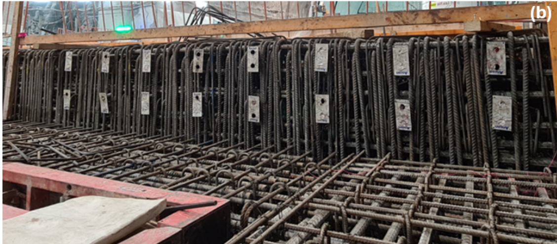
Figure 8. Capping Beam reinforcement details.
