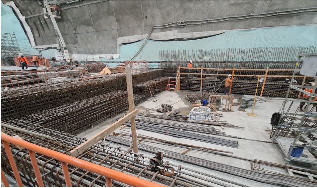
Figure 7. Kicker and capping beam assembled reinforcement
