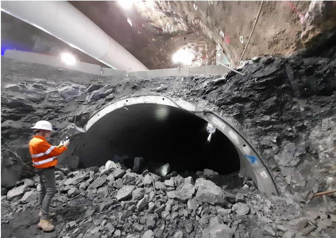
Figure 2. Breakthrough into the segmental lining showing the nominal cover over the crown (16 December, 2021)
