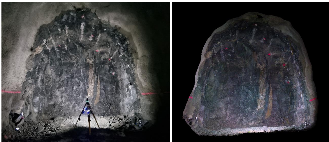
Figure 4 TLS capture of a drill and blast tunnel excavation (left) with corresponding georeferenced point cloud output (right)
