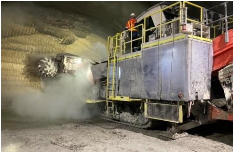
Figure 1. Sandvik MT720 Roadheader excavating rock.
