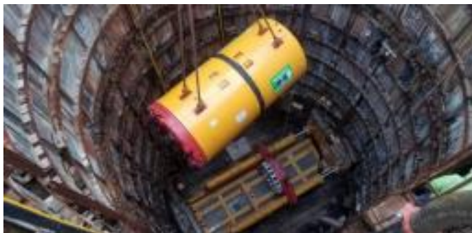
Figure 6. AVN1500 lowered into launch shaft for 1,203 meters record drive in Painesville, Ohio.
