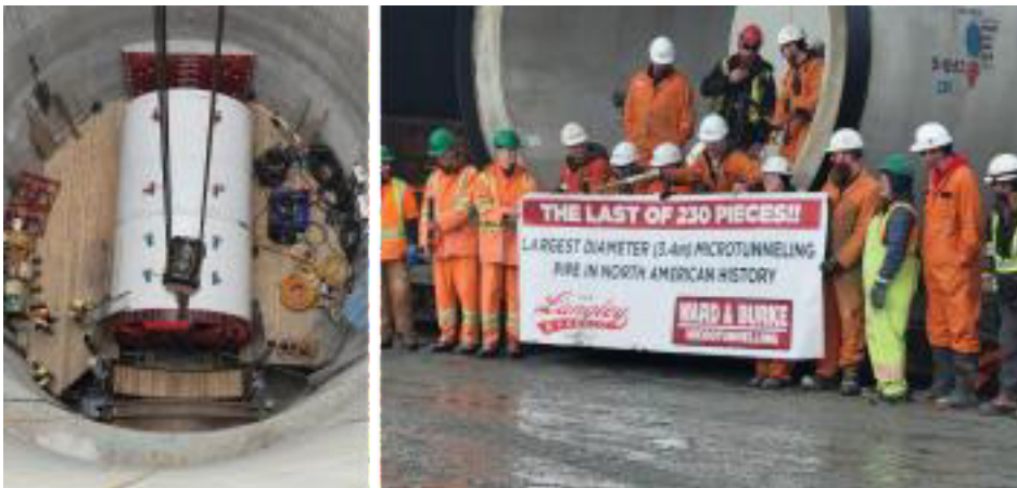
Figure 9. Launch shaft and breakthrough ceremony on North America's largest diameter pipe jacking jobsite (© Ward & Burke).
