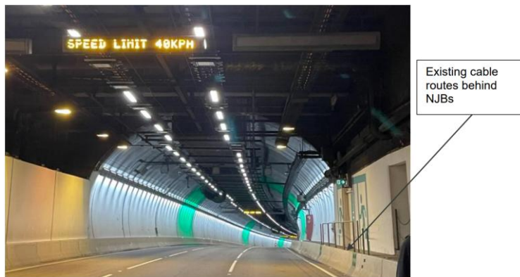
Figure 3. Burnley Tunnel existing cable routes' location.
