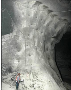
Figure 1: Pillar covered by wiremesh and bolts to prevent sudden brittle failure (Esterhuizen et al., 2011)
