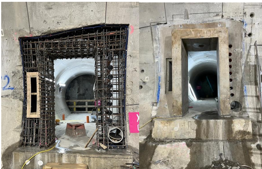
Figure 9: Cross passage reinforcement and concrete after striking
