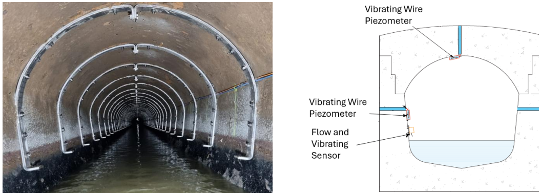
Figure 9 – Left: Sewer Strapping, Right: Sewer Lining I&M arrangement
