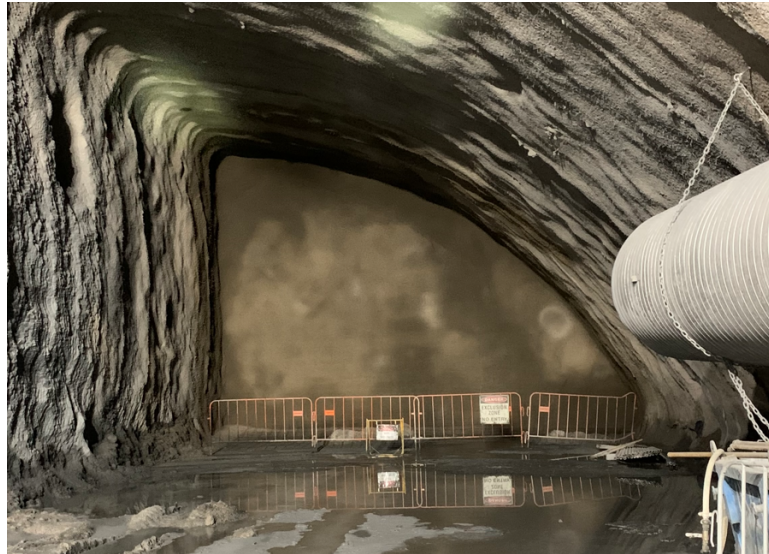
Figure 3. Typical signage and barrier set up in cavern
