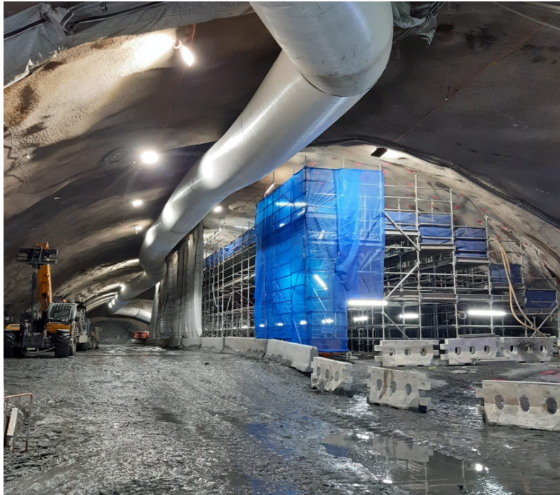
Figure 8. Scaffold erection in constrained top heading
