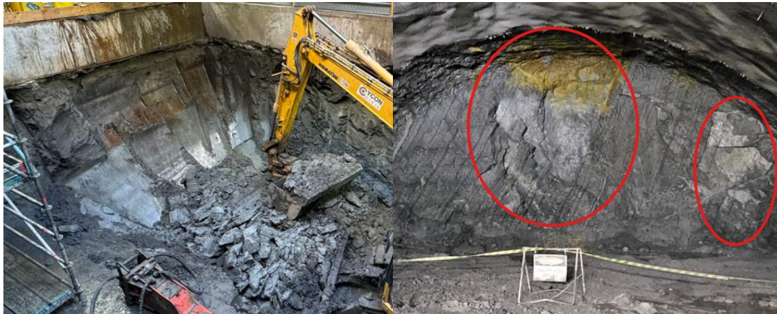
Figure 2. Inferred hydrothermally altered rock with clay-like strength in the northbound portal excavation (left). Inferred hydrothermally altered rock with decreased strength from surrounding rock in heading excavation denoted by red circles (right).
