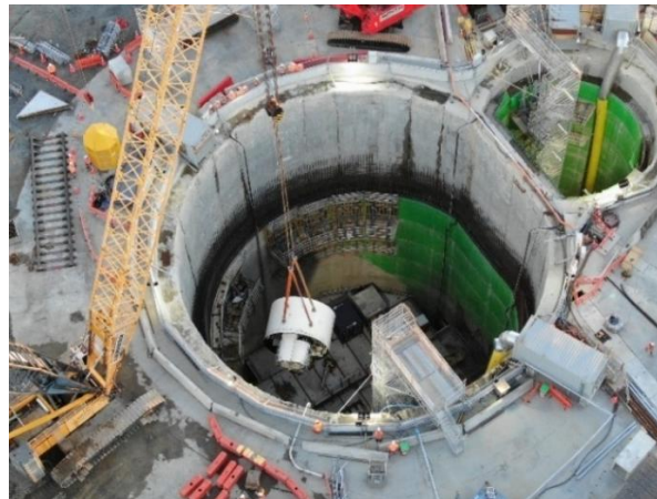
Figure 4. MPS shafts during TBM launch, PE corrosion protection lining is green.
