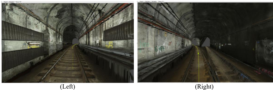
Figure 4. 3D reconstruction of tunnel lining using Dibat8 software. (Left) Colour-mapped mesh of the Down Track tunnel surface. (Right) Crown region showing darker-coloured 2004 shotcrete overlay compared to the original 1971 lining.
