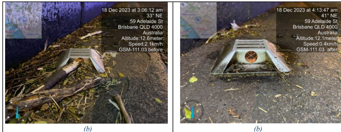
Figure 4. (a) Debris found on cats eye prism in the gutter post rain. (b) Cleaned following maintenance
