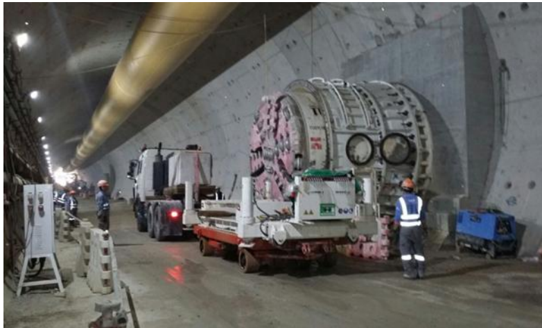
Figure 5. AVN 3000 recovery in the tunnel, after breakthrough into reception bell
