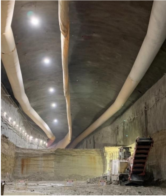
Figure 5. Sandvik Mt720 roadheader excavating a deep bench in ventilation cavern VF02
