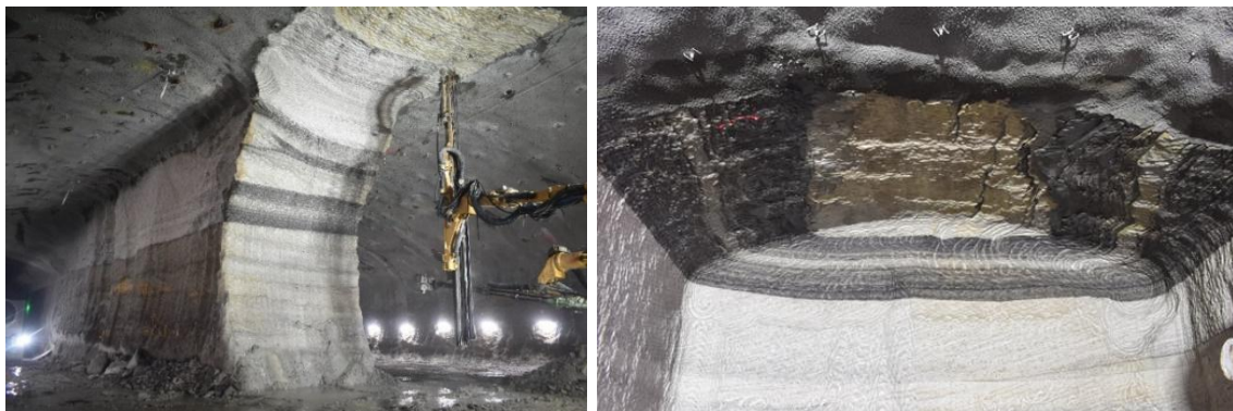
Figure 10. Laminite band in Cavern 1 temporary pillar (top heading 3) (left) and adjacent M150 ramp (right).
