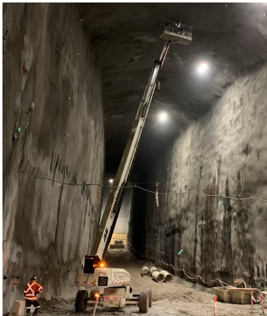
Figure 4. Inspection of endoscope hole for monitoring of rock bolts shearing in crown of completed ventilation cavern.
